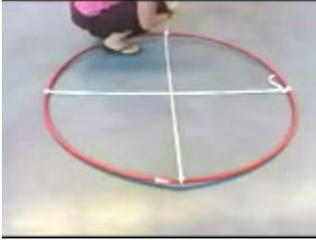
1. Take a segment of medium rope about 10 ft long. Fold it in half and tie it across the circle at two of the marked points opposite each other. Repeat for the other two marks with another length of rope. [Optional: the ropes can be duct taped where they meet the frame to prevent sliding during construction.]
