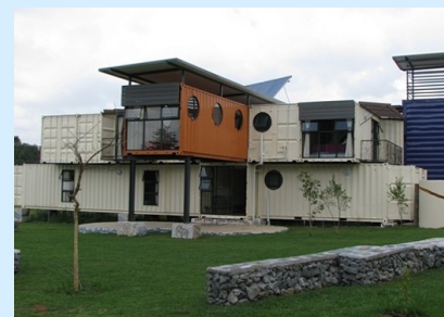
The Children's Home building is made from used shipping containers.
