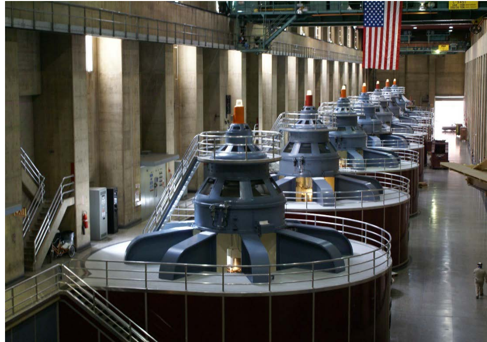
Generators inside the Hoover Dam. Magnets are pushed through a coils of wire. Image Credit: Richard Martin CC 2.0
