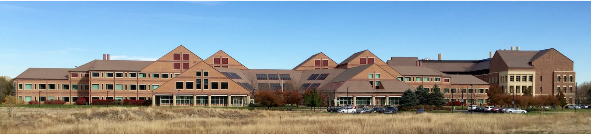
Sustainability, Energy and Environment Community (SEEC) Building
